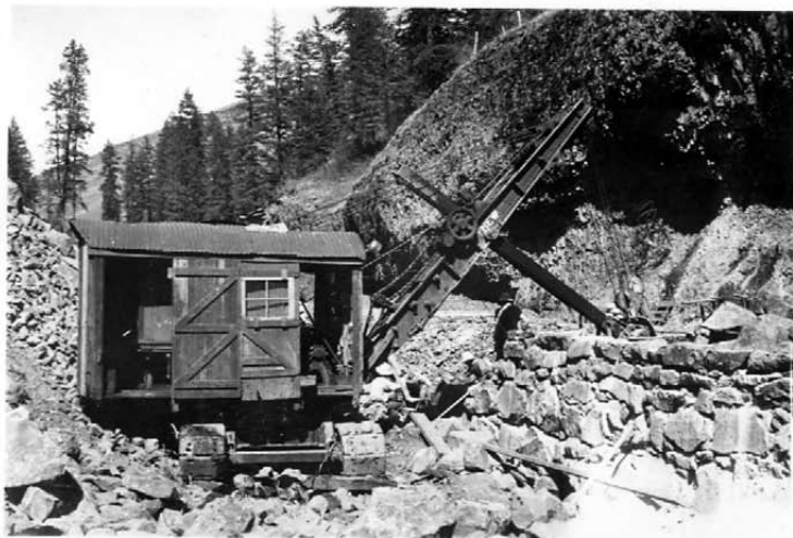
No. 48. WPA 3/8 CY The Shovel used as crane when building Ruble Wall Station 365400. August 1937.
